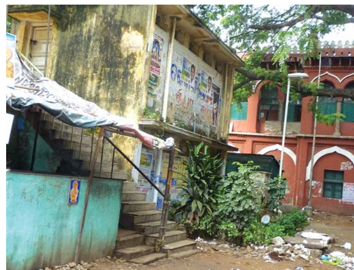
A permanent toilet block.
