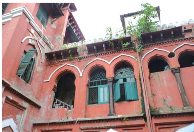
Tree growth has a field day at Chepauk Palace with its broken windows and what fills in for them when they have vanished.
