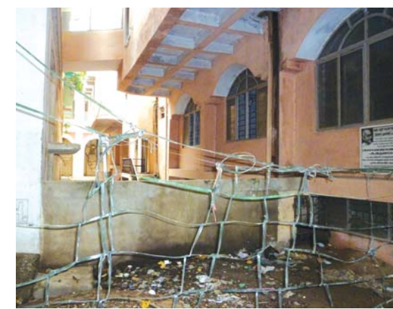
New buildings that have come up to completely shut out the palace. Note the tangle of wires.
