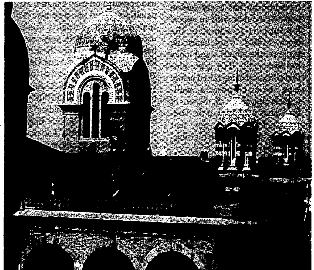
Restoring the roof is the first priority at Senate House.
