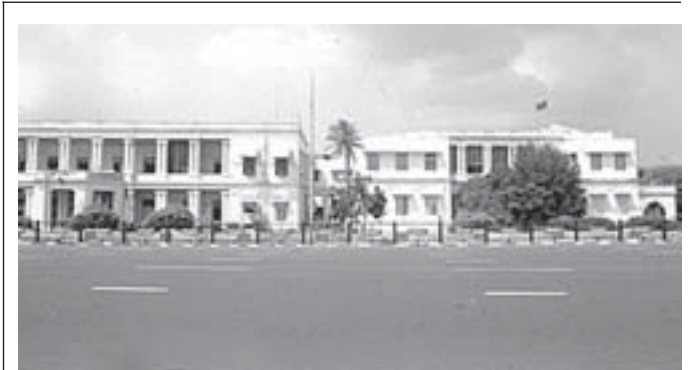
The restored DGP building on the Marina.
