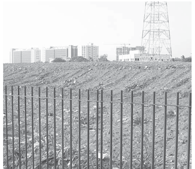
Raising of embankment in progress along the Adyar.
