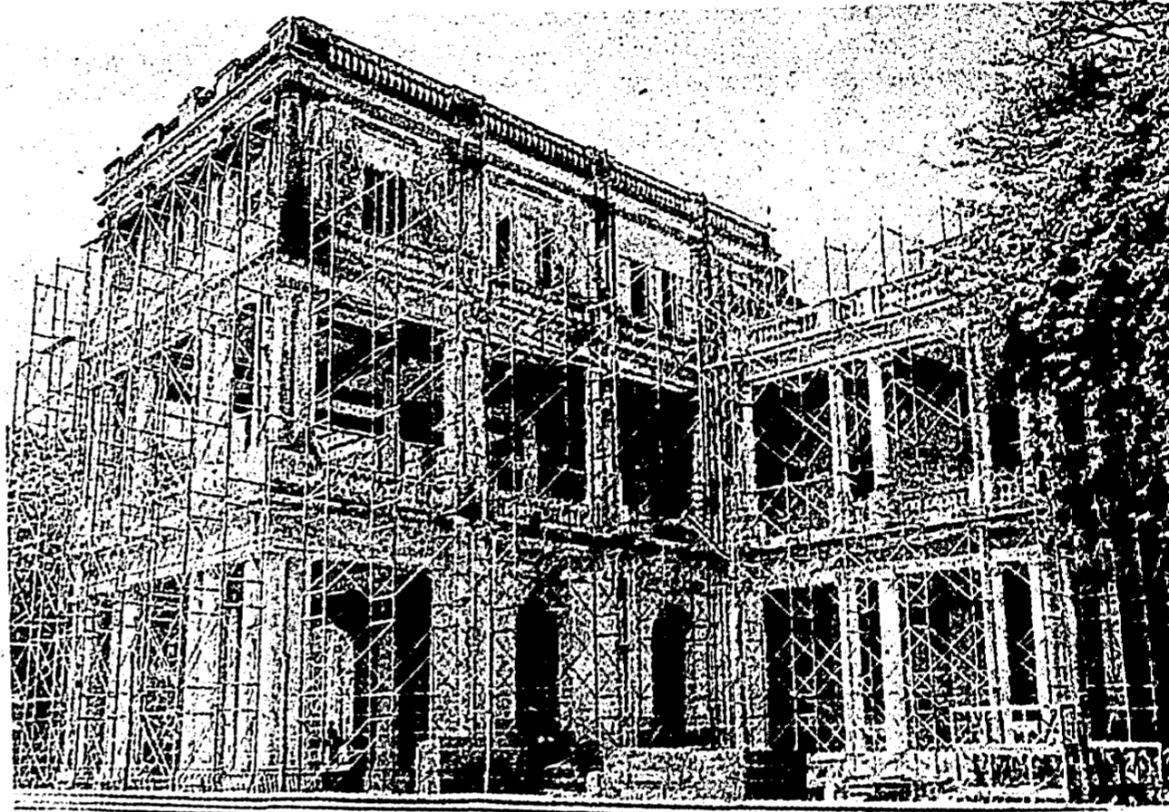
Sprucing up Government House in Government Estate.
