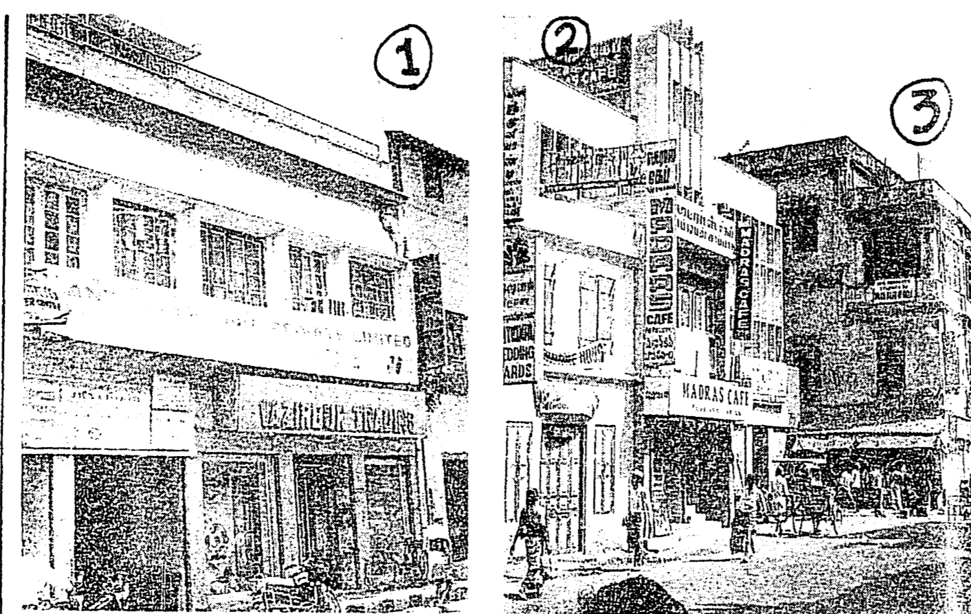
Researching another project, Rajind Christy came across the rather striking old building on the right, discovered that it was 8 Popham's Broadway. It had been the offices of the Madras Times from 1901 to 1909. It was owned by Gantz, Pere et Fil, then the leading printers in Madras. Following through, Christy came with the other photographs we feature in this rather unusual OLD and NEW.
